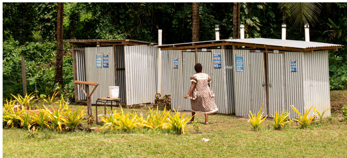
Bangabulu School's improved facilities, which are single-sex for students and teachers and include handwashing facilities, Red Cliff, South Ambae, Vanuatu.
