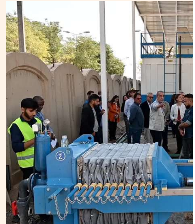
UNICEF and the United Nations Assistance Mission for Iraq (UNAMI) collaborated to install an MBBR wastewater treatment system at the UNAMI office building. MBBR systems installed across Iraq help reduce water shortages worsened by climate change. ©UNICEF Iraq
