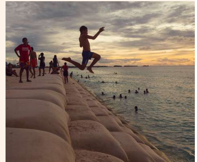
Liveti, 12, jumps from a sandbag staircase in Tuvalu that was built by the government to combat rising sea levels. The structure, called The Reclaimed Land, spans 78,000 m 2 – around 780 m long and 100 m wide – and is fortified on three sides with robust sandbags to hold back the ocean. ©UNICEF/UNI560974/Bak Mejlvang
